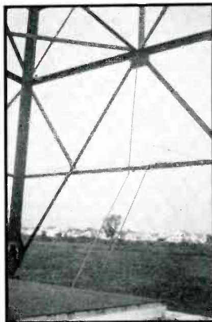
FIG. 7—The a-m line, at the right, terminates at the first tower-brace. A copper bond runs around the tower at this point. The f-m line continues up the tower
