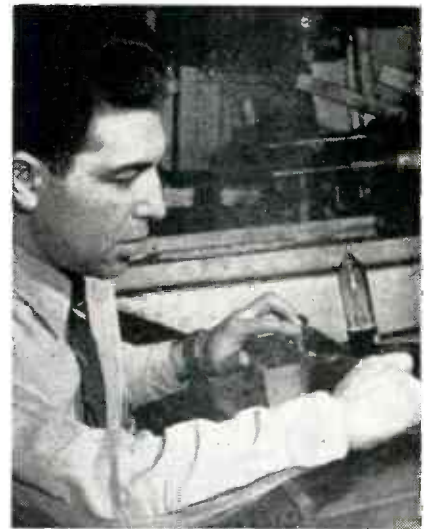
A vacuum-tube thermocouple, that anticipates temperature changes of an electric furnace, is adjusted by its inventor, M. J. Manjoine of Westinghouse Research Laboratories
